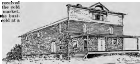
2410. A storage house in western New York, built with particular reference to storing apples.
